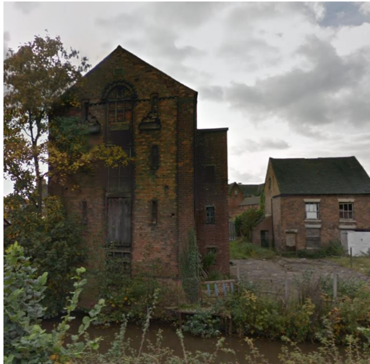
Figure 3: Photo of the old Mill building along the canal.
