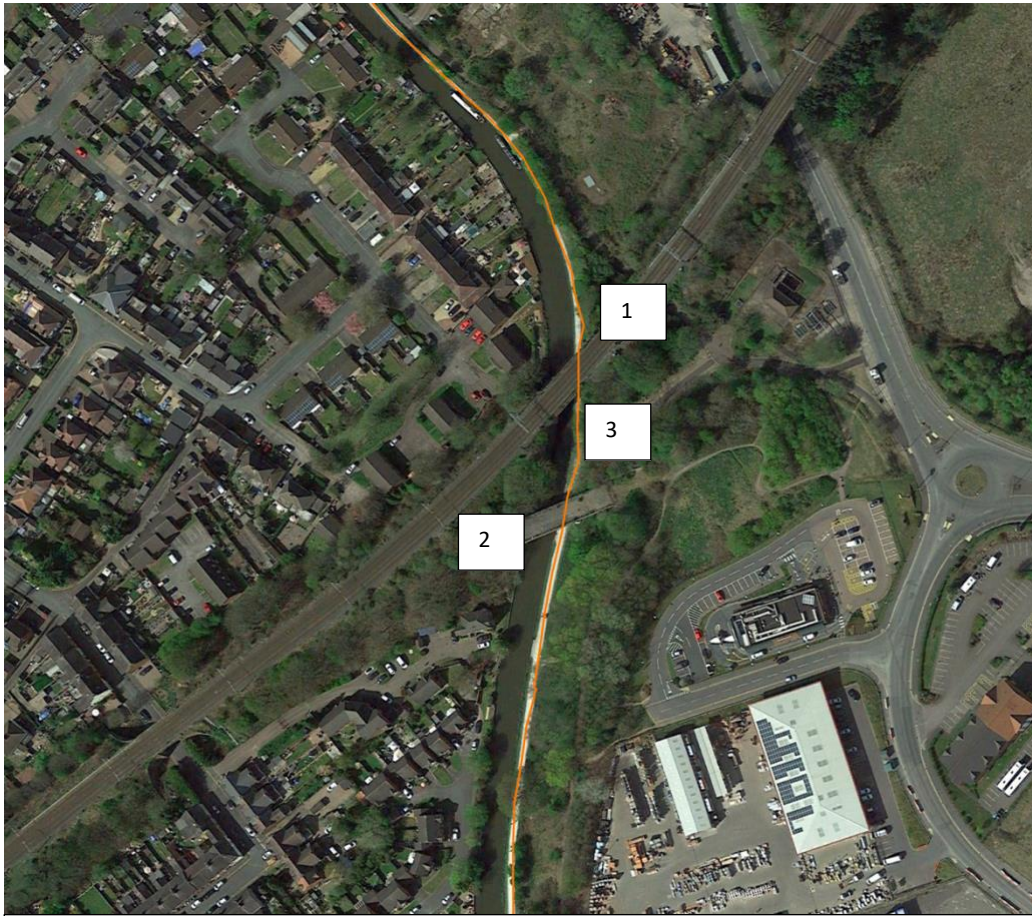
Figure 4: Aerial image of the two railway bridges and canal.
