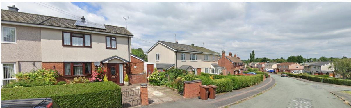
Figure 4 – Properties in Springfield Avenue, predominantly semi-detached solid wall properties, aging from 1930-1960
