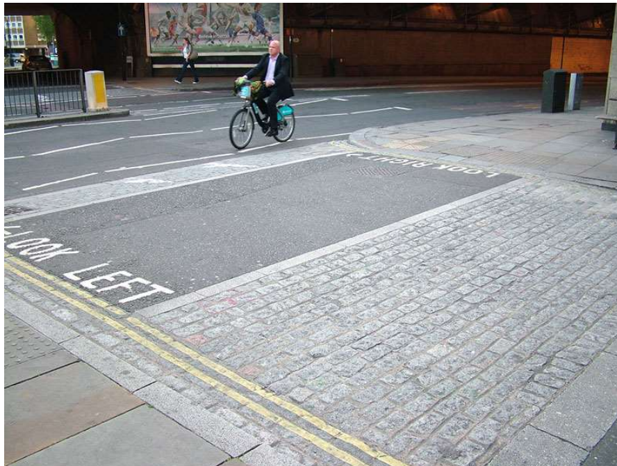
Figure 10: UK example of raised, uncontrolled crossing point of a side road (source: 'The Alternative Department for Transport' website) 6
