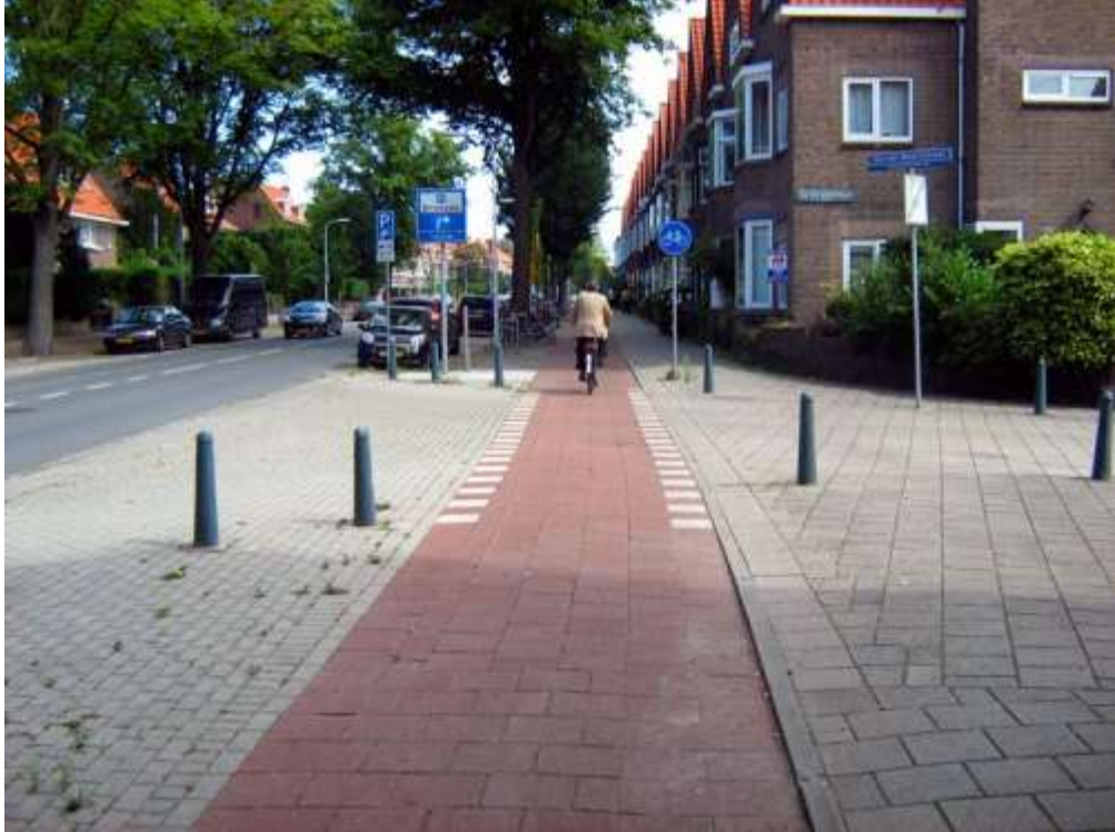
Figure 11: Example of raised, uncontrolled crossing point of a side road (source: 'The Alternative Department for Transport' website) 6
