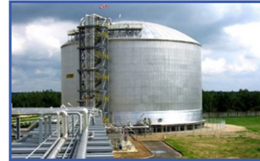
AB Achema 15,000T Ammonia Storage Tank, Lithuania. Source: Thyssenkrupp Industrial Solutions
